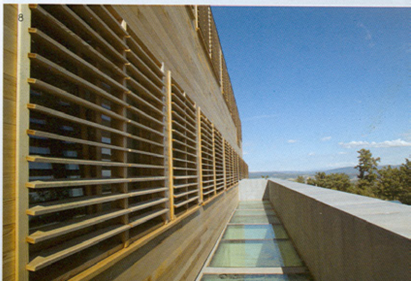
5. 6. 7. 8. The Monastery of Siloe
